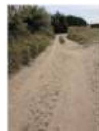
Between Car Park and Manor Road
